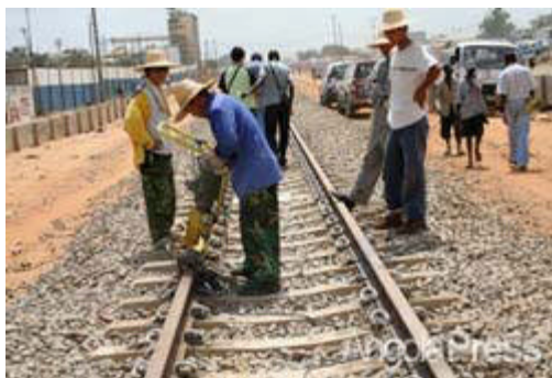
Luanda railway rehabilitation works
